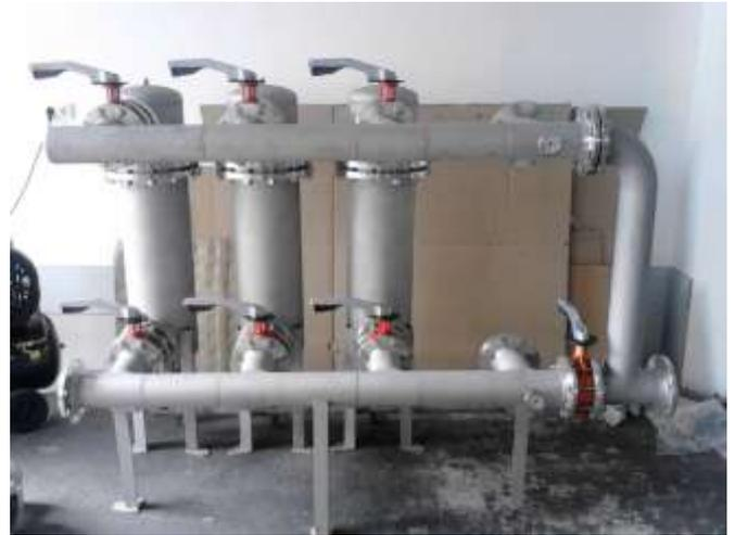
**Name:** Thermal water filtering system (95°C warm water) for district heating
