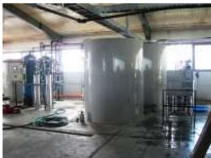
Complete filtering system with gravel bed and reverse osmosis in the tire industry
